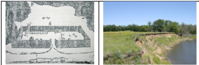
A sketch made by Hartney historian Larry Clarke and the site today.
